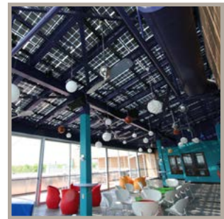
Moonrise Hotel, St. Louis image courtesy of Microgrid Solar
